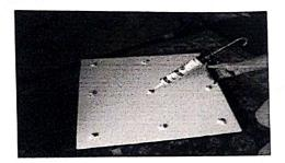
Construction adhesive is a general-purpose adhesive used for attaching drywall, tile, molding, and fixtures to walls, ceilings, and floors. It is most commonly available in tubes intended for use.
