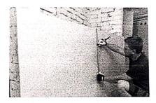
Plasterboard is a panel made of calcium sulfate dihydrate (gypsum) usually pressed between a facer and a backer. It is used to make interior walls and ceilings. This 'Drywall' construction became popular as a quicker alternative to traditional lath application.
